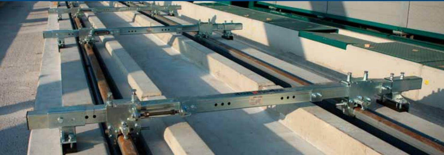
Installation and geometric alignment of the rails take place in accordance with the two techniques described below (Top-Down and Bottom-Up). For the embedding work, either project-dedicated machines pour the Corkelast®, or it is applied by manual pouring from buckets.
